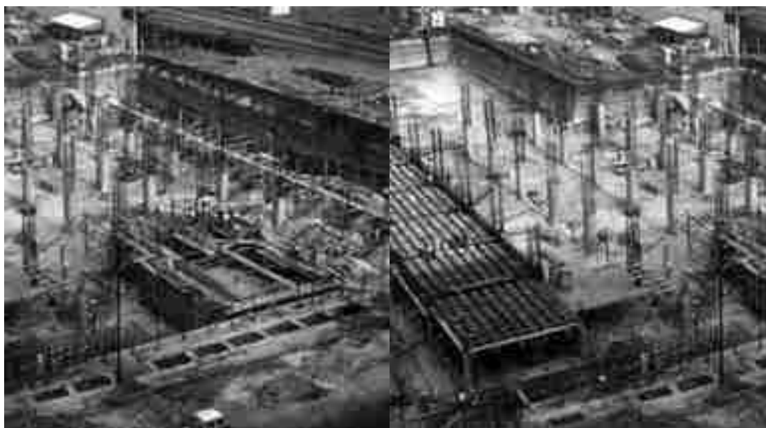
Figure 2.11. Construction of Credito Hipotecario building (Gatonelblu, 2010)
