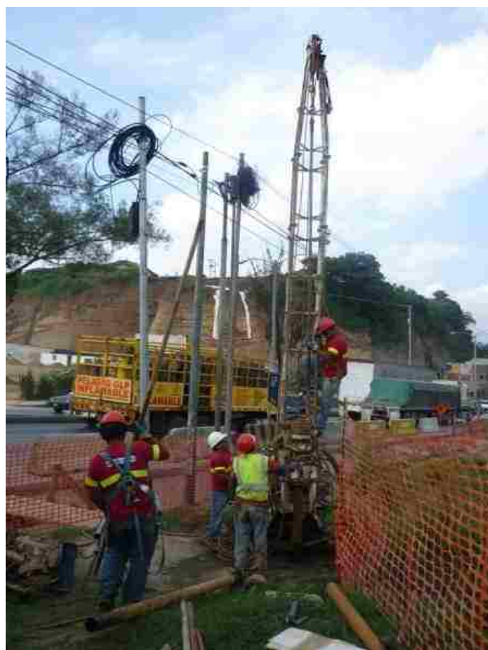
Figure 4.5. Boreholes drilling
