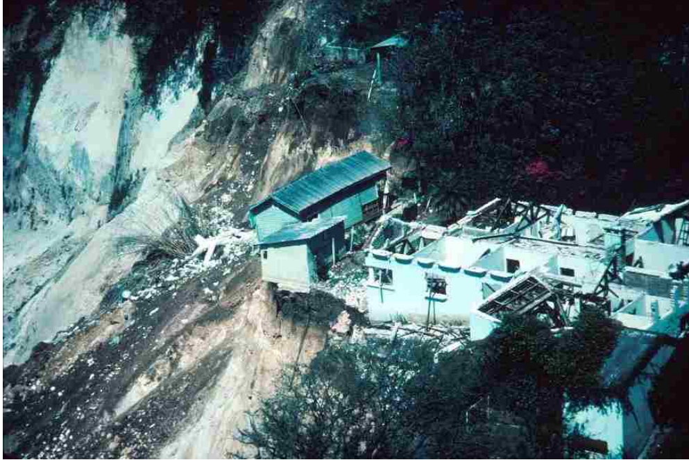
Figure 2.5. Landslide along the edge of a steep walled valley in Guatemala City (Plafker, 1977)
