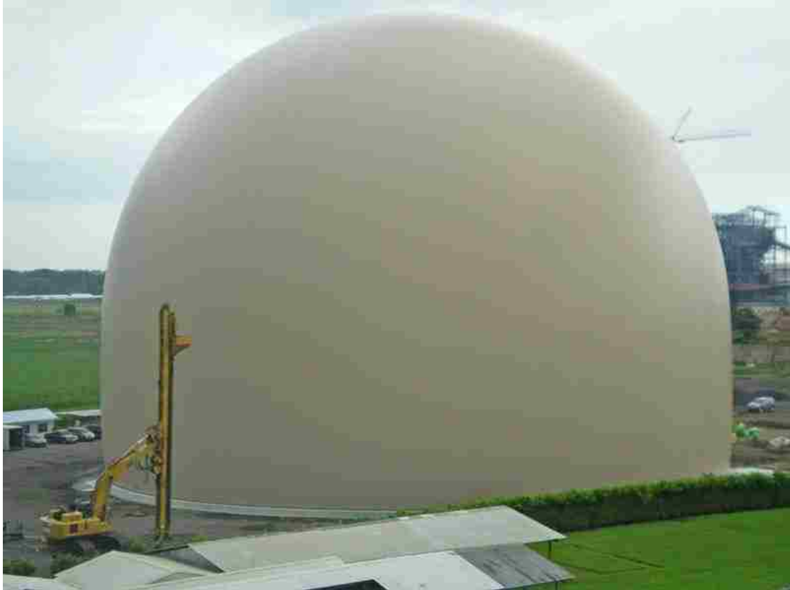
Figure 2.22. Magdalena Sugar Storage Facility (Soiltec, 2012)
