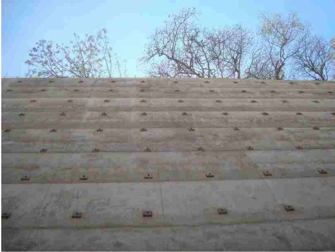
Figure 3.1. Vertical soil nailing wall for excavation stabilization
