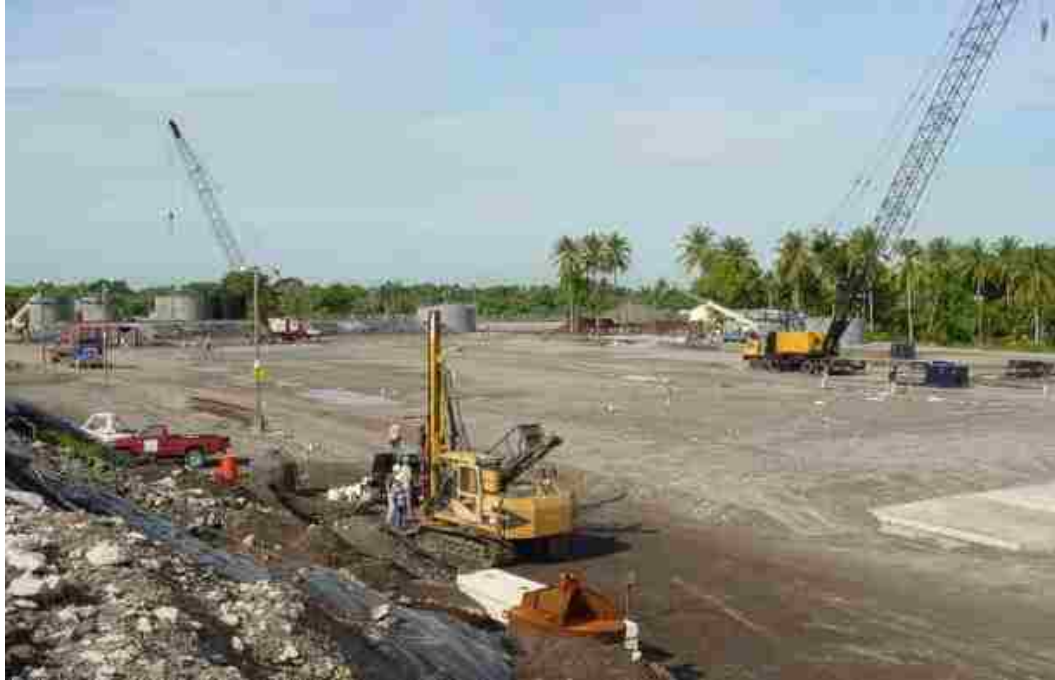
Figure 2.13. Construction site of Arizona Power Plant
