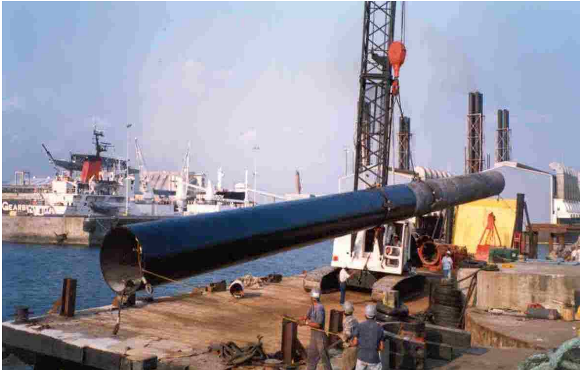
Figure 2.15. Steel piles of Barcaza Man
