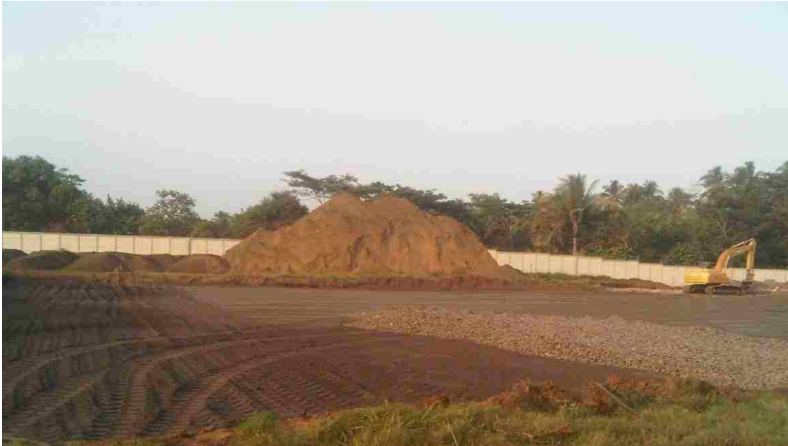
Figure 4.52. Working platform construction
