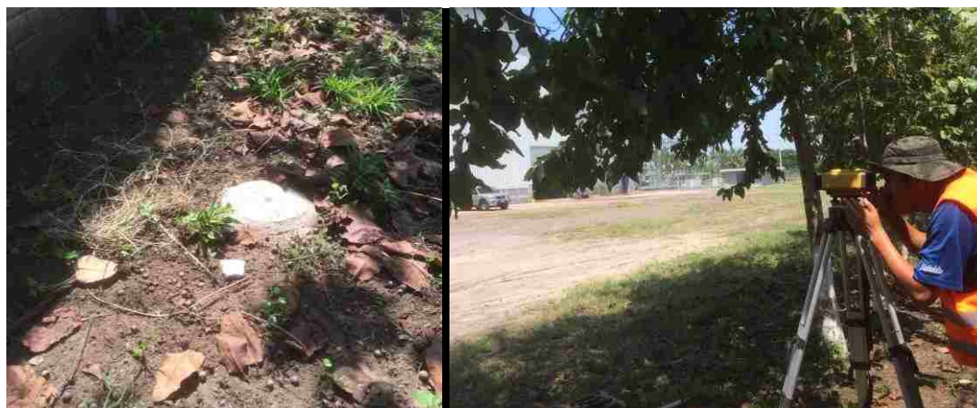
Figure 4.66. Survey monument and surveying works
