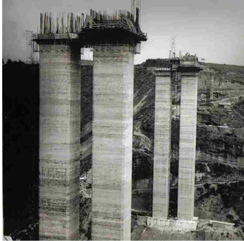
Figure 2.18. Construction of Incienso Bridge piers (Rodas, 2012)
