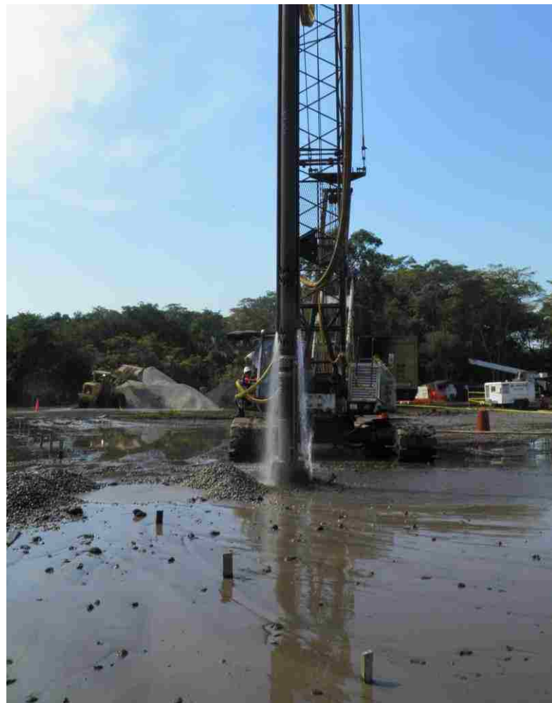
Figure 4.53. Vibroflot penetration
