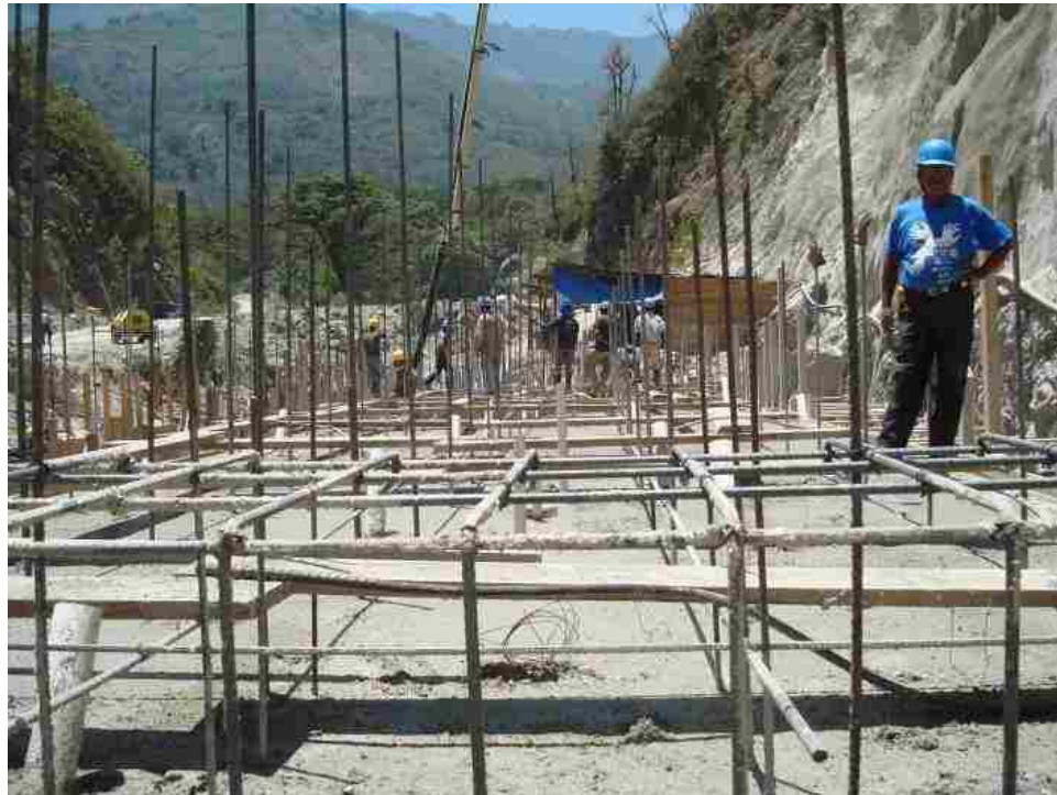
Figure 4.28. PVC sleeves intalled during construction
