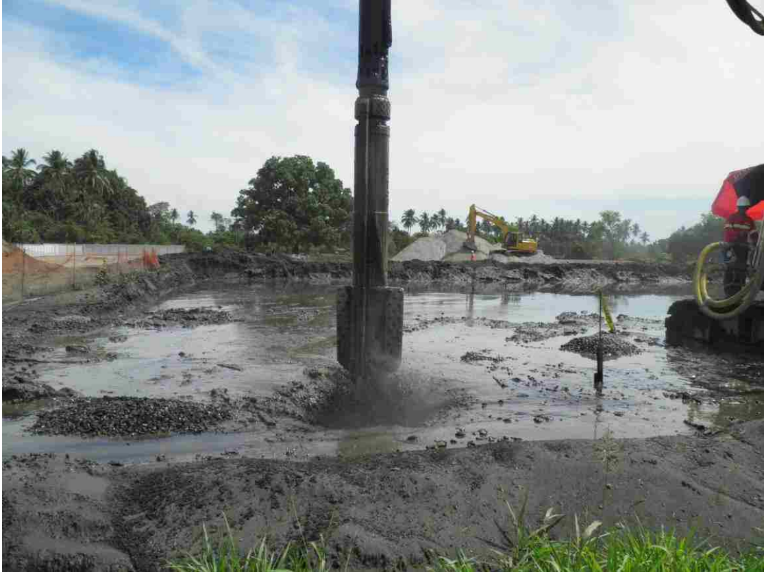
Figure 4.55. Final stage of the compaction process
