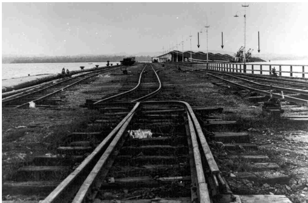
Figure 2.9. Puerto Barrios wharf, destroyed by the February 4 earthquake. Arrows point to the large warehouse partially submerged ((Plafker, 1977)
