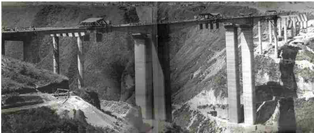
Figure 2.17. Construction of Incienso Bridge deck (Castillo, 2009)
