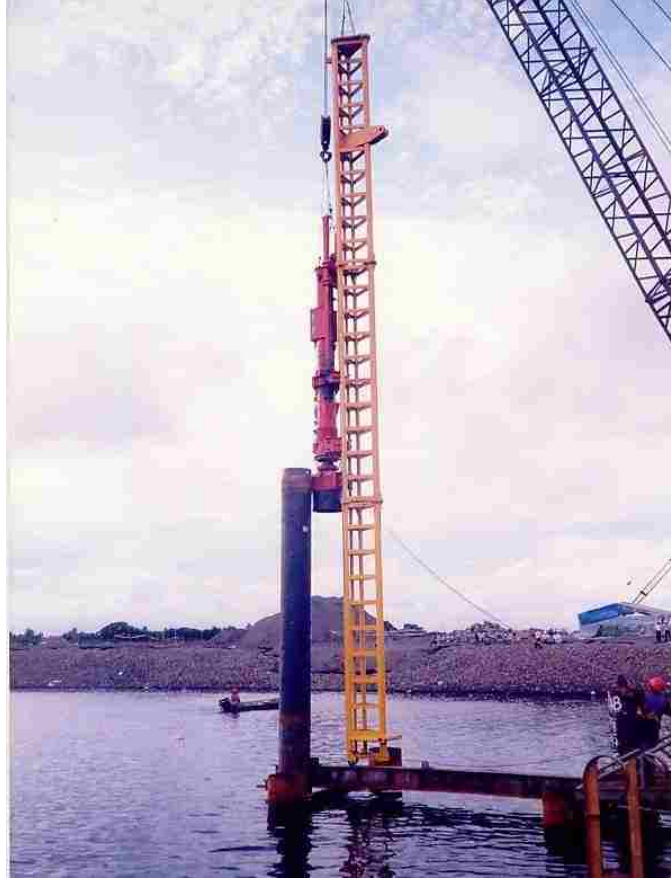
Figure 2.16. Construction of San Jose Docking Station
