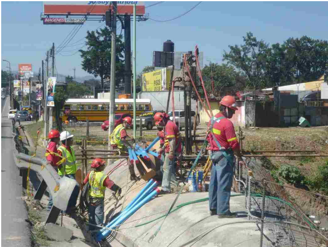
Figure 4.14. Inclinerometer installation
