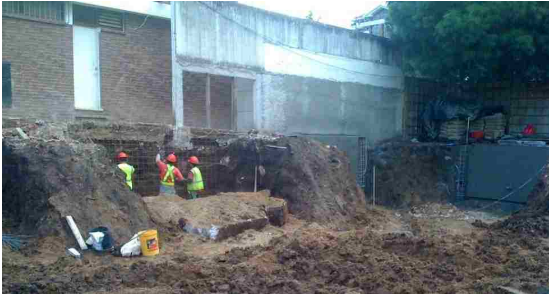
Figure 3.2. Berm utilization during construction
