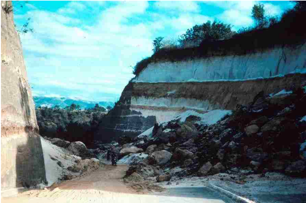
Figure 2.6. Landslides in steep roadcut of stratified pumice and ash deposits at San Cristobal (Plafker, 1977)
