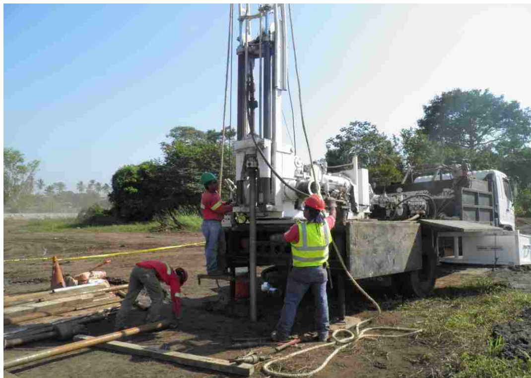
Figure 4.44. Borehole drilling using rotary core system
